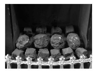
f) Select three of the medium sized coals and arrange along the fuelbed behind the second row of large coals, as shown below in Fig. 6
