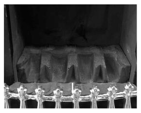
c) Fit six of the medium sized coals onto the front ceramic rail, ensuring that they are evenly spaced. Use the recess's in the front ceramic rail as a guide for placement. (See fig. 3 below)
